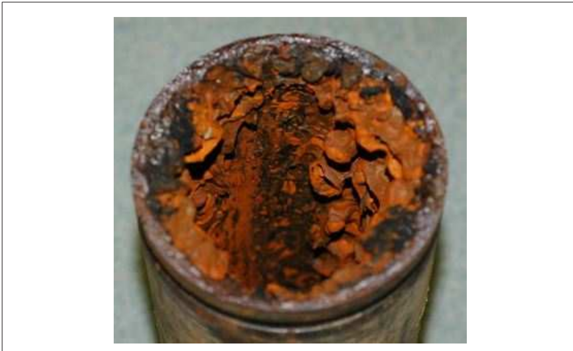
Fig. 15. Corroded steel pipe with many tubercles inside
