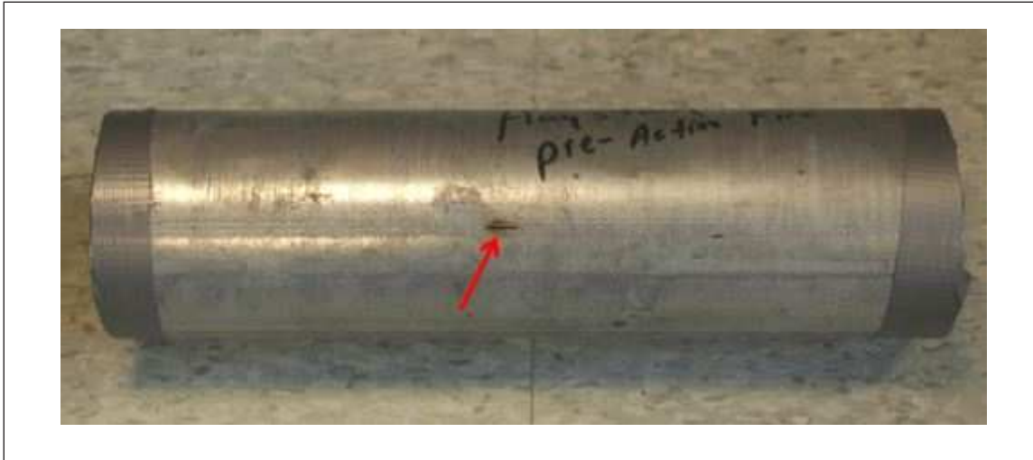
Fig. 13. Grooving corrosion of a longitudinal through-wall leakage in a galvanized steel pipe along its weld seam in a preaction
