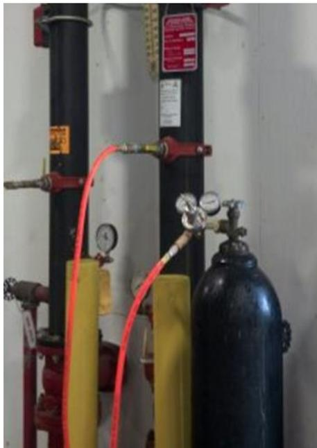
Pressurized cylinders provide nitrogen gas through injection ports at risers
