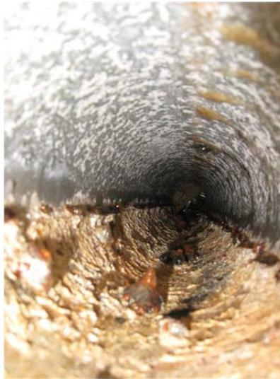
**Evidence of trapped water in piping**
