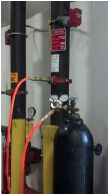
Pressurized cylinders provide nitrogen gas through injection ports at risers
